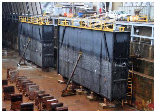
Testing the operation of 2 new caissons in Gatun Spillway.
